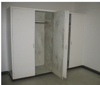
Poor Indoor Air Quality and Mold Evident Throughout Unoccupied Portion of Building
