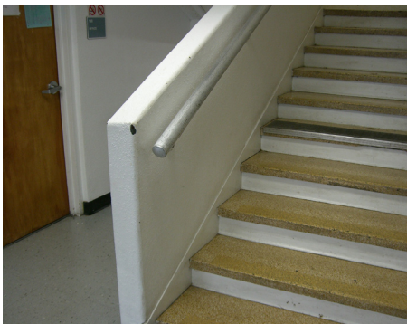
Stair Handrails and Guardrails are Not Compliant
