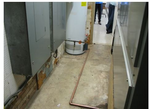
No Code Required Clearance in Front of Electrical Panels
