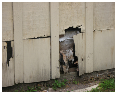
Exterior Wall Rotted and in Very Poor Condition
