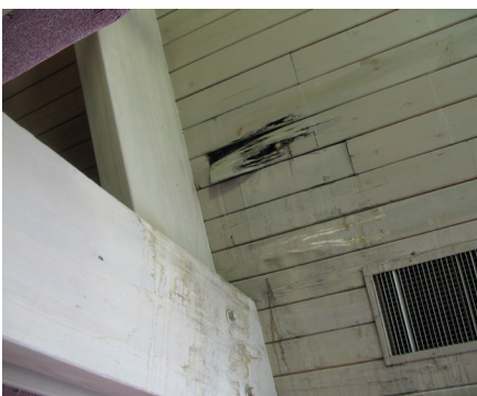
Deterioration at Wood Siding
