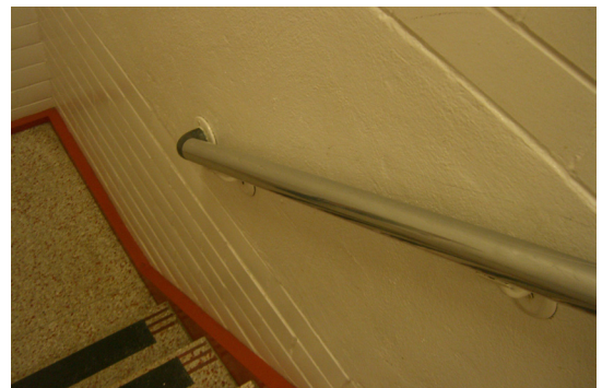
Handrails Not ADA Compliant
