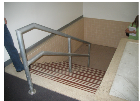
Handrails/Guardrails Not ADA Compliant
