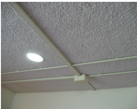
Electrical Run in Surface-Mounted Conduits
