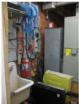
Electrical Mixed in with Mechanical and Mop Sink
