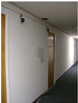
Patch in Wall and Base in Disrepair
