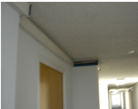
Electrical Run in Raceway
