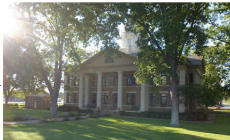
Mason County Courthouse
